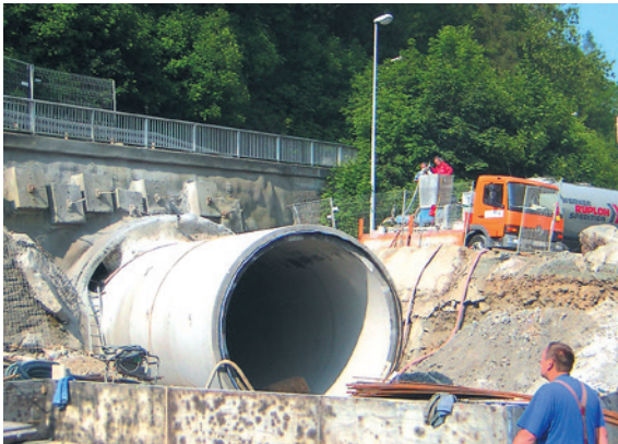
Backfilling of annular spaces
