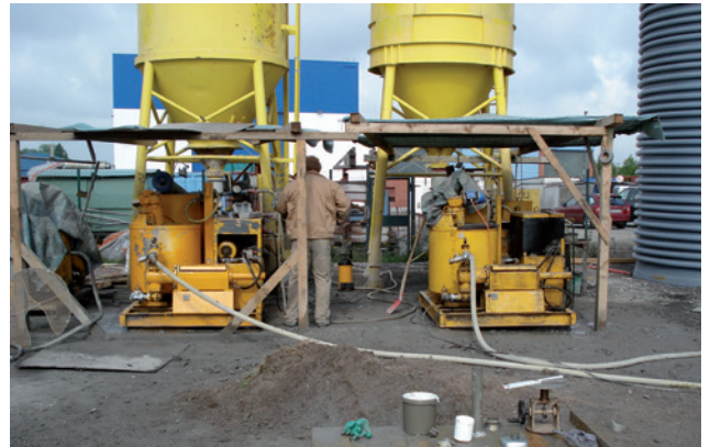
Cavity backfilling
