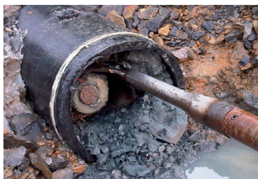
← Removal of the cable with a special drilling head
