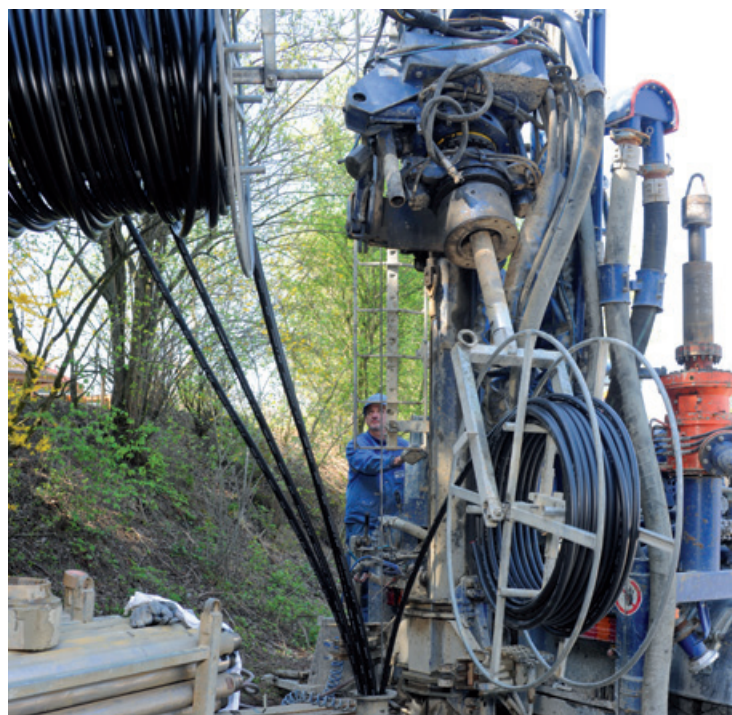
Installation of geothermal probe incl. injection pipe. →
