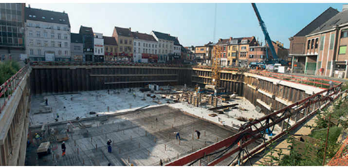
← Finished construction pit: CSM wall with inserted sheet pile wall
