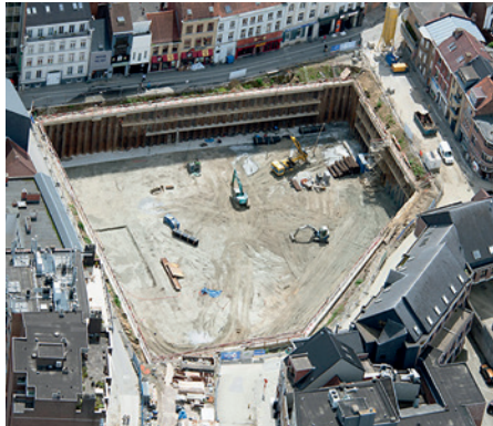
↑ The finished construction pit: CSM wall with inserted sheet pile wall
